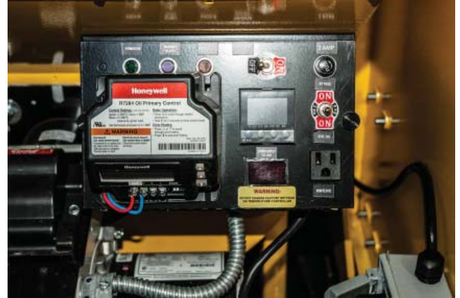
Heater Control Panel
