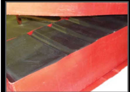
Full Environmental Spill Containment around poly tank
