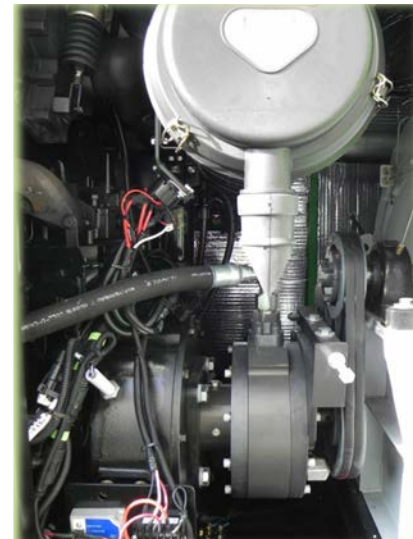
Interior from the Right Side of the Unit Front Door
